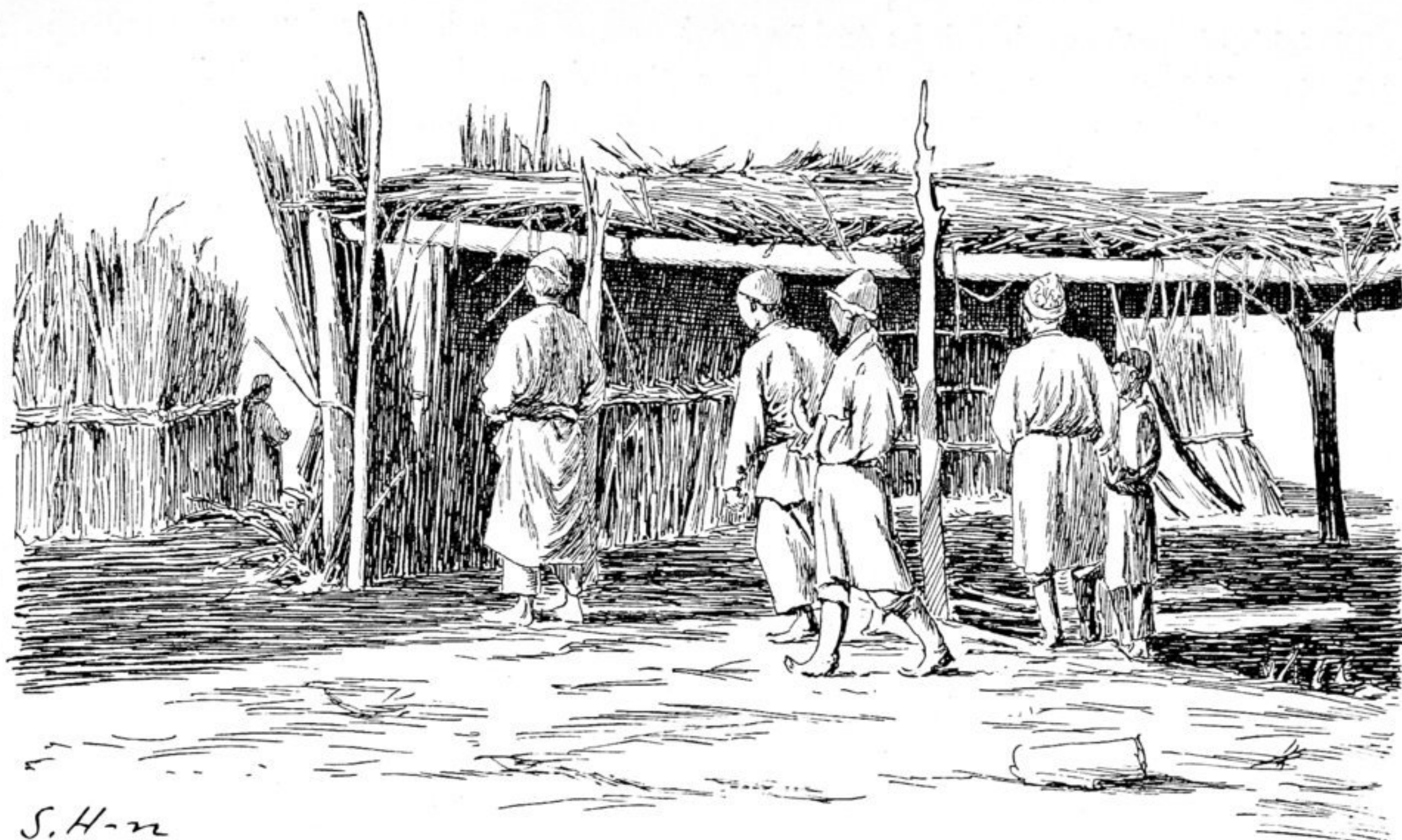
Fig. 120. THE UJ HALF FINISHED.
