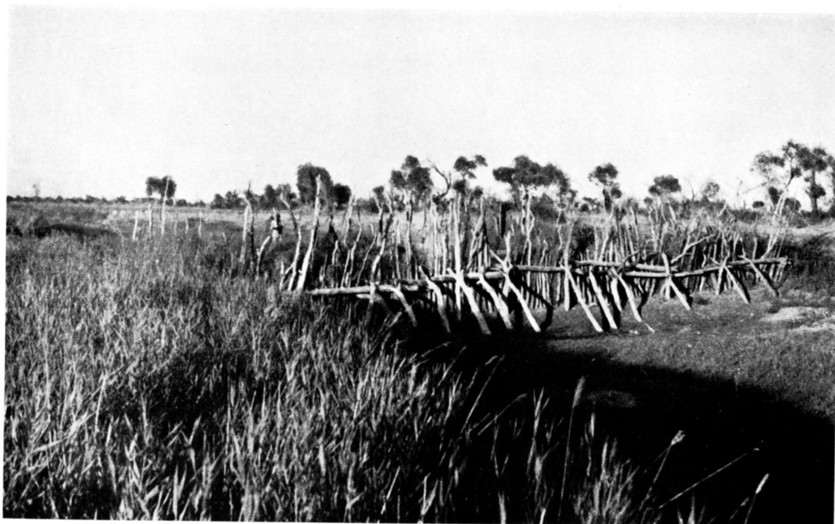
Dam-structure in the old bed of the Konche-darya at Temenpu, built to prevent the water from flowing into the new bed of the Qum-darya. Compare map Fig. 7
