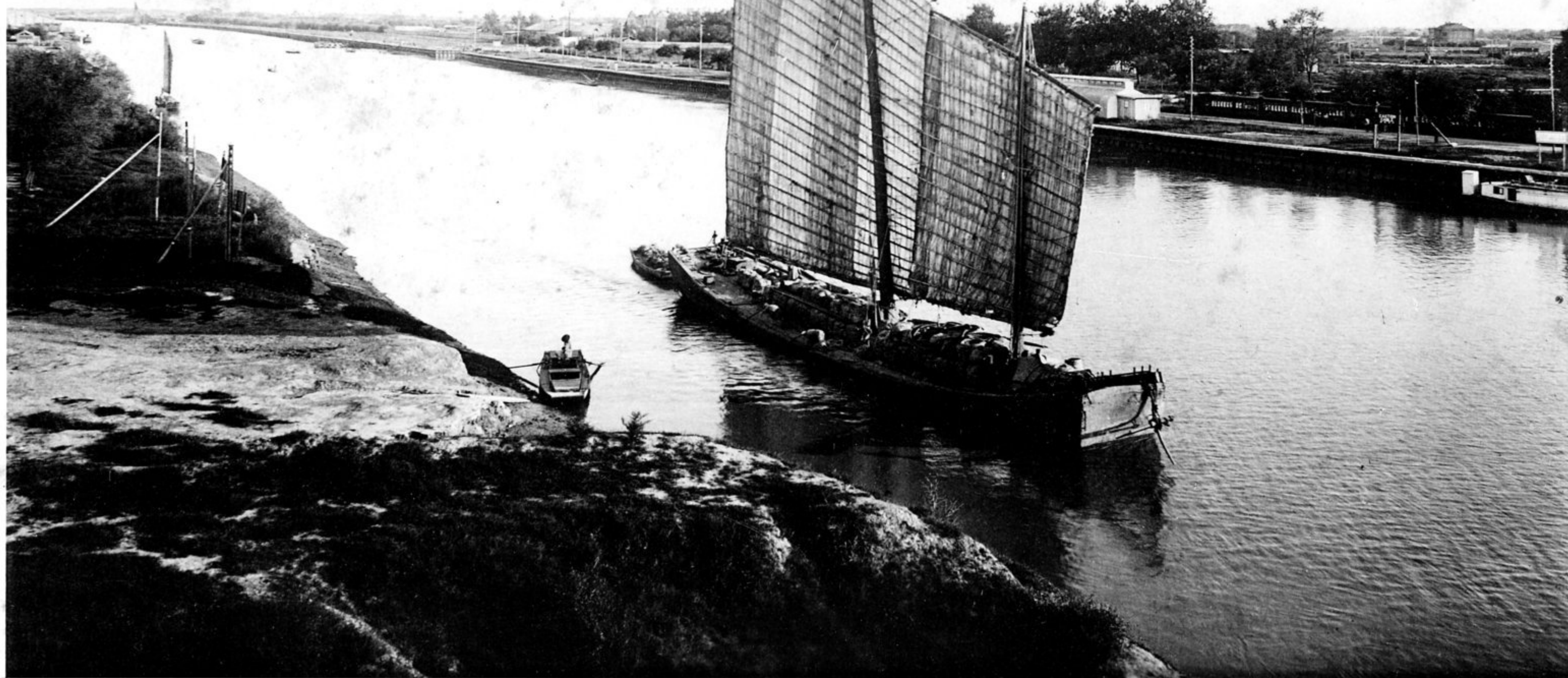
リナ部一ノ界租逸獨ハ岸對所ルストンラ、カニ街市ノ地留居津天ニ將テシ航溯回迂ヲ折曲ノ餘有十七河白 岸沿ノ界租逸獨（河白）（津 天） (Tien Tsin) The River Paiho. The entrance of the Tien Tsin Port, the opposit Bund is a part of the German Concession.
