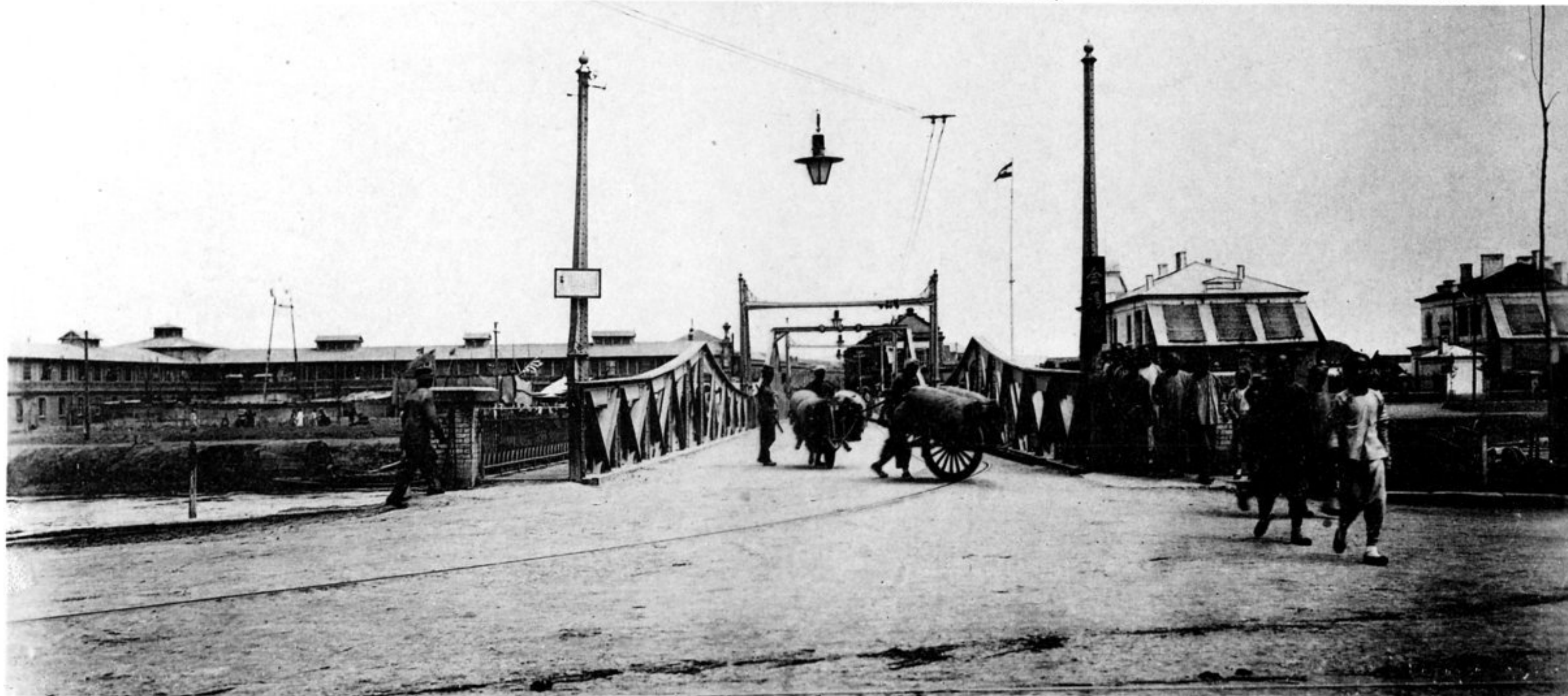
リナ組仕ル得ヲトコルス閉開在自リヨ央中メ爲ルムシセ過通ヲ船民テシニ橋鐵ルス接連ヲト界租國澳ト街市那支 橋湯金 (津天) (Tien Tsin) Chin Tang Bridge. This is built across the River Paiho between Australian Concession and Chinese City.
