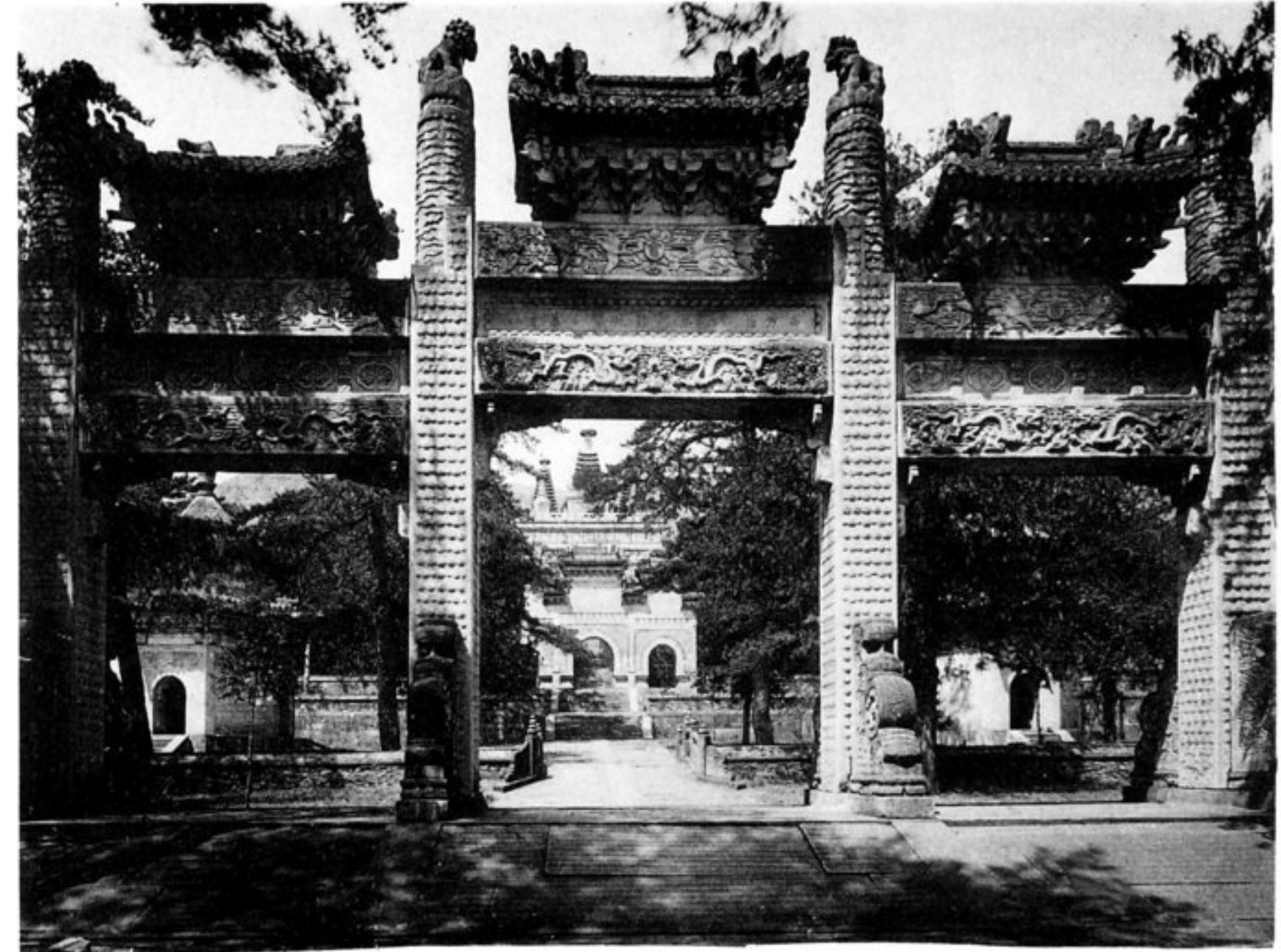
リアニ地ノ里六約トコル距ヲ門直西ノ京北アシニ立建ノ賢忠魏朝明 寺雲碧 Pi-Yun Temple, 3 miles from Peking. This was erected during Ming dynasty.
