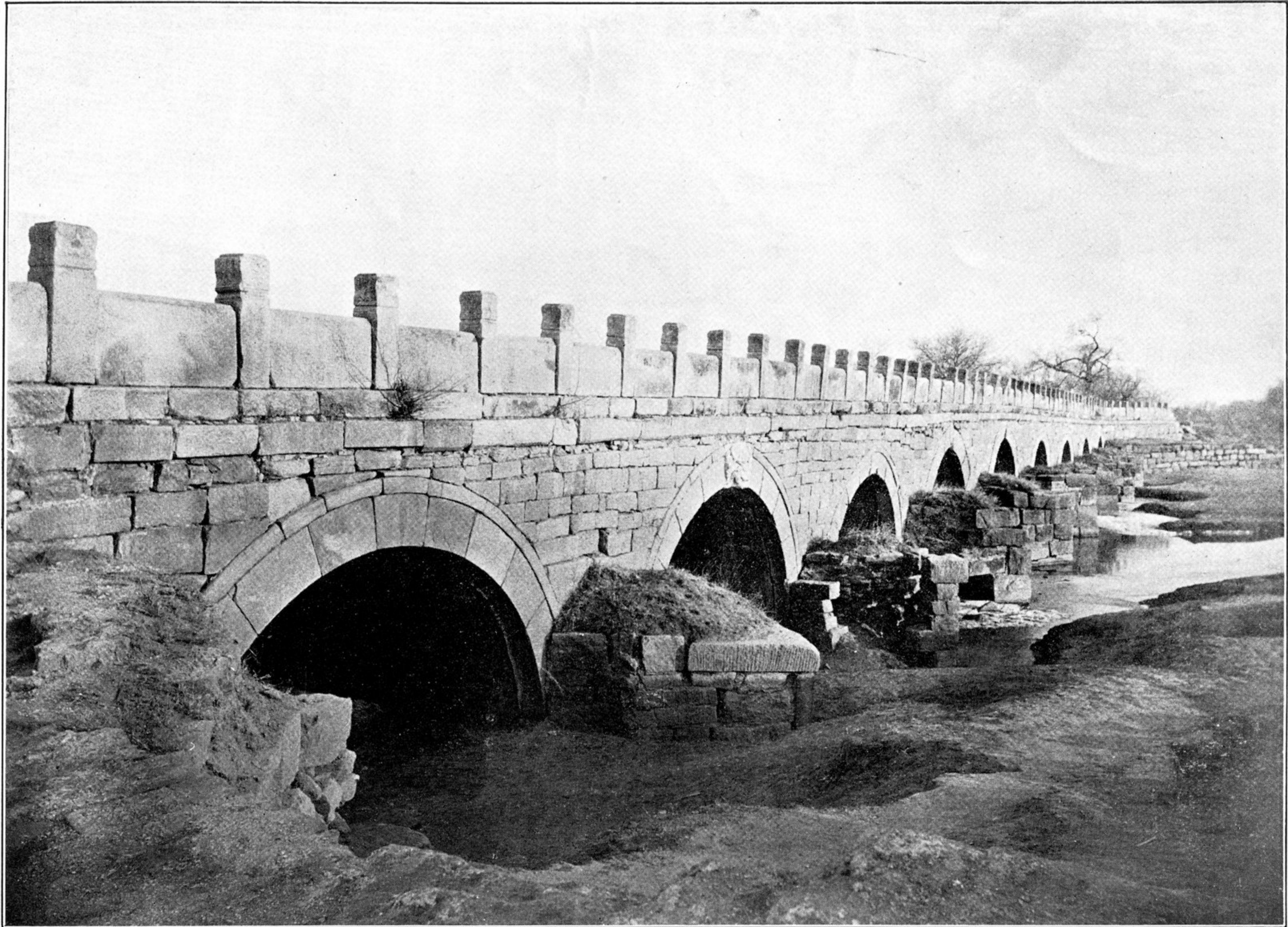
No 52. Sha-Ho-ch'iao Bridge.
