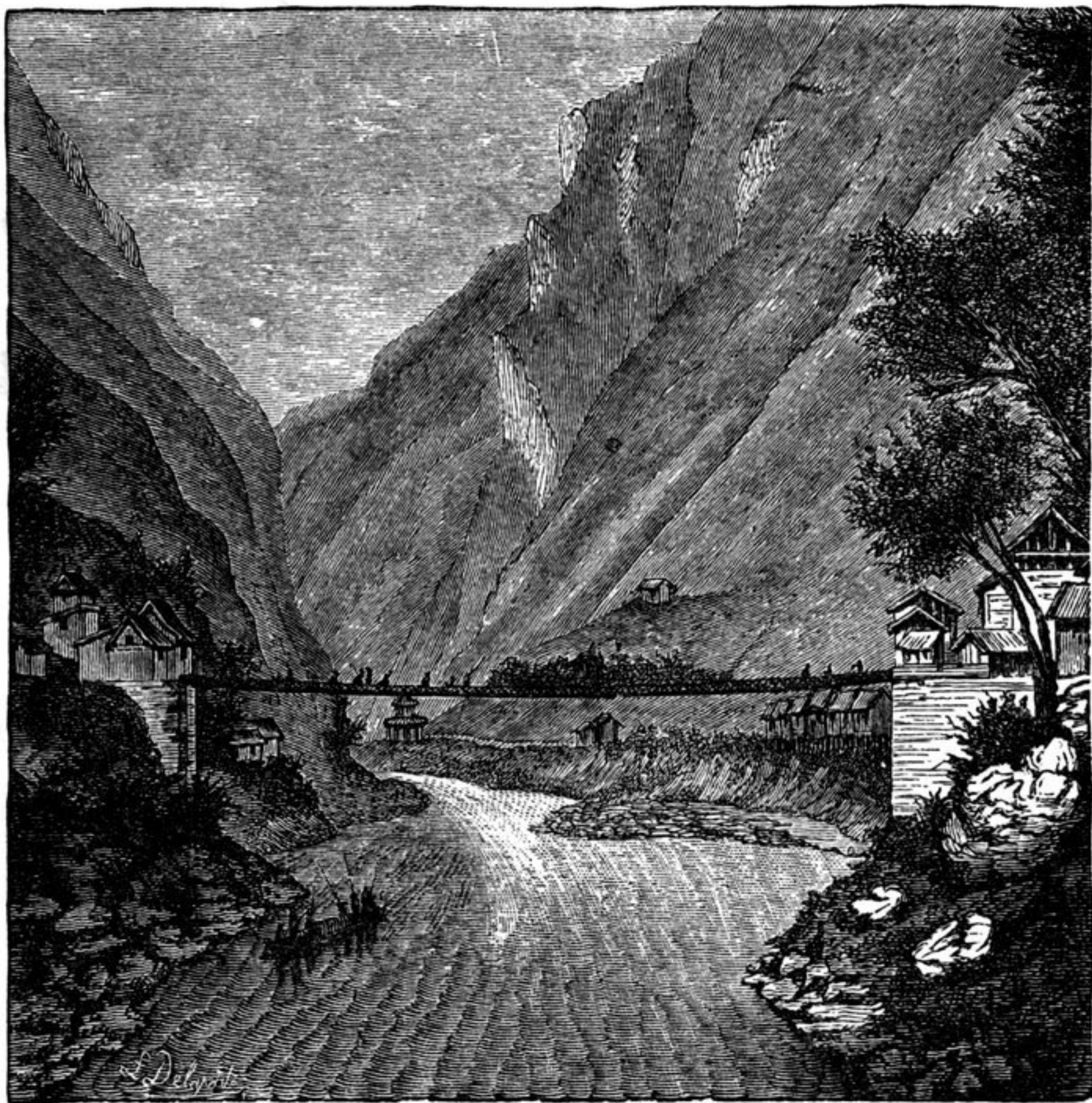
Iron Suspension Bridge at Lowatong. (From Garnier.)
