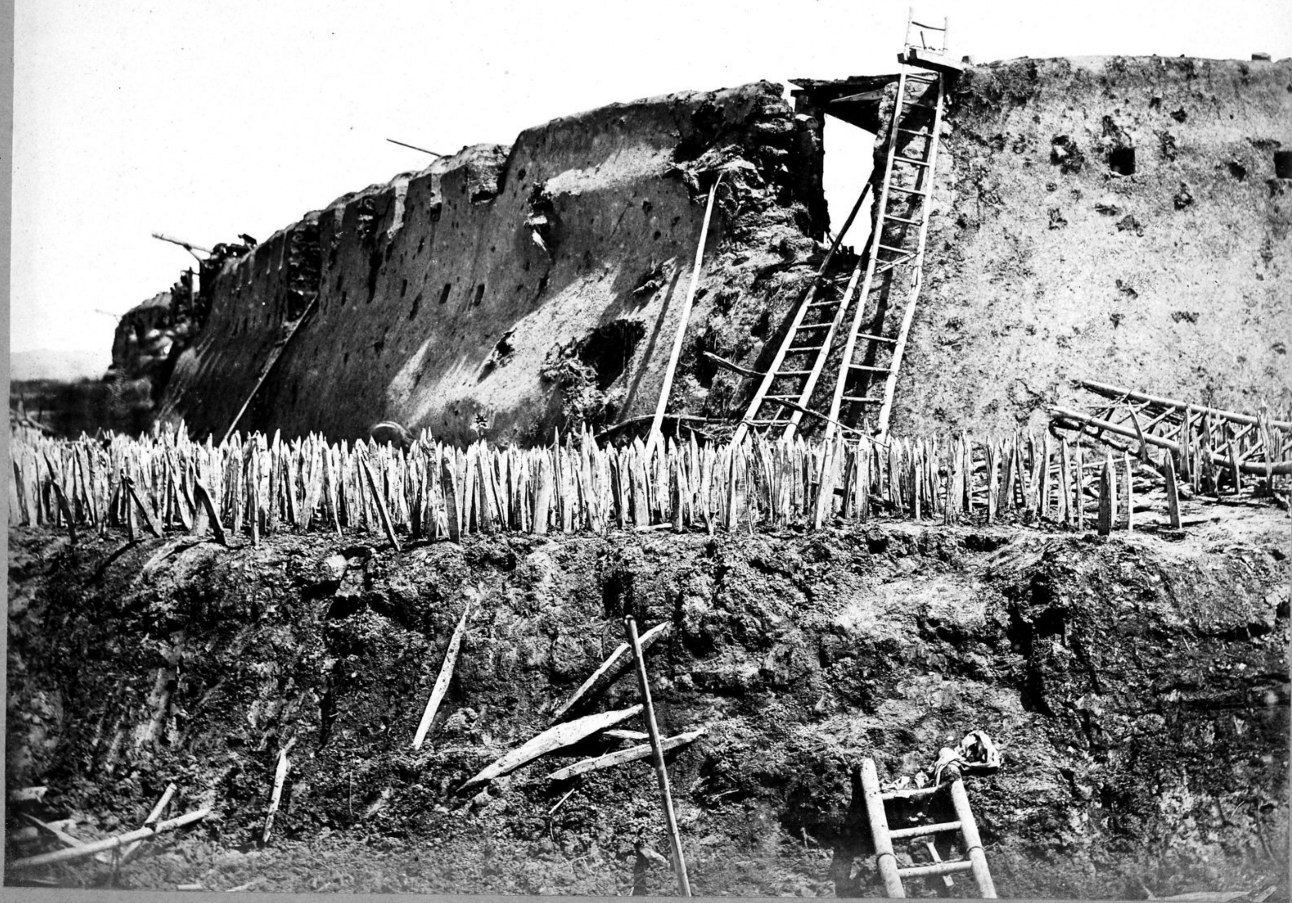
Angle of the North Fort. Showing where the French entered. Aug. 21/60.
