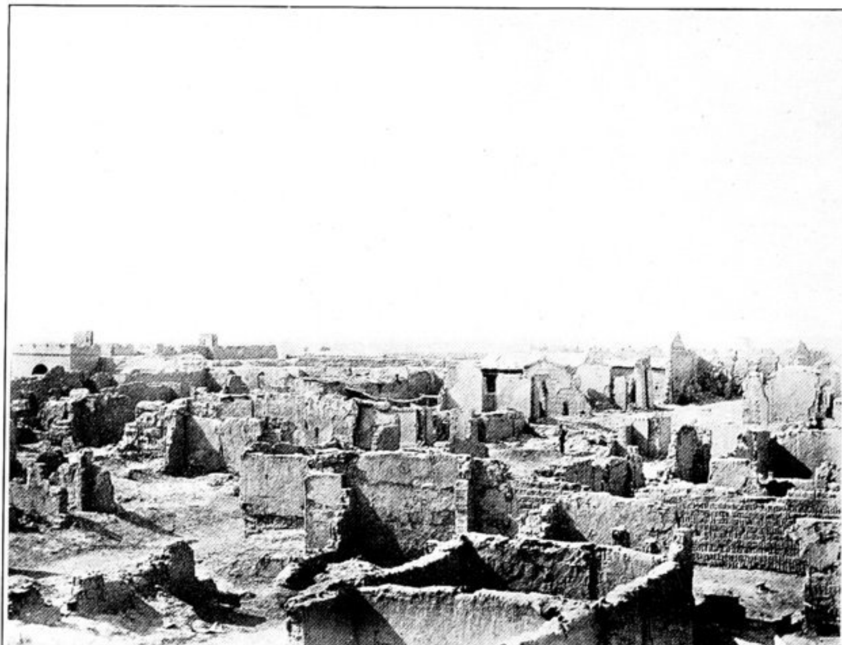
217. INTERIOR OF RUINED FORTRESS CH'IAO-WAN-CH'ÉNG ON LIMES EAST OF BULUNGIR.
