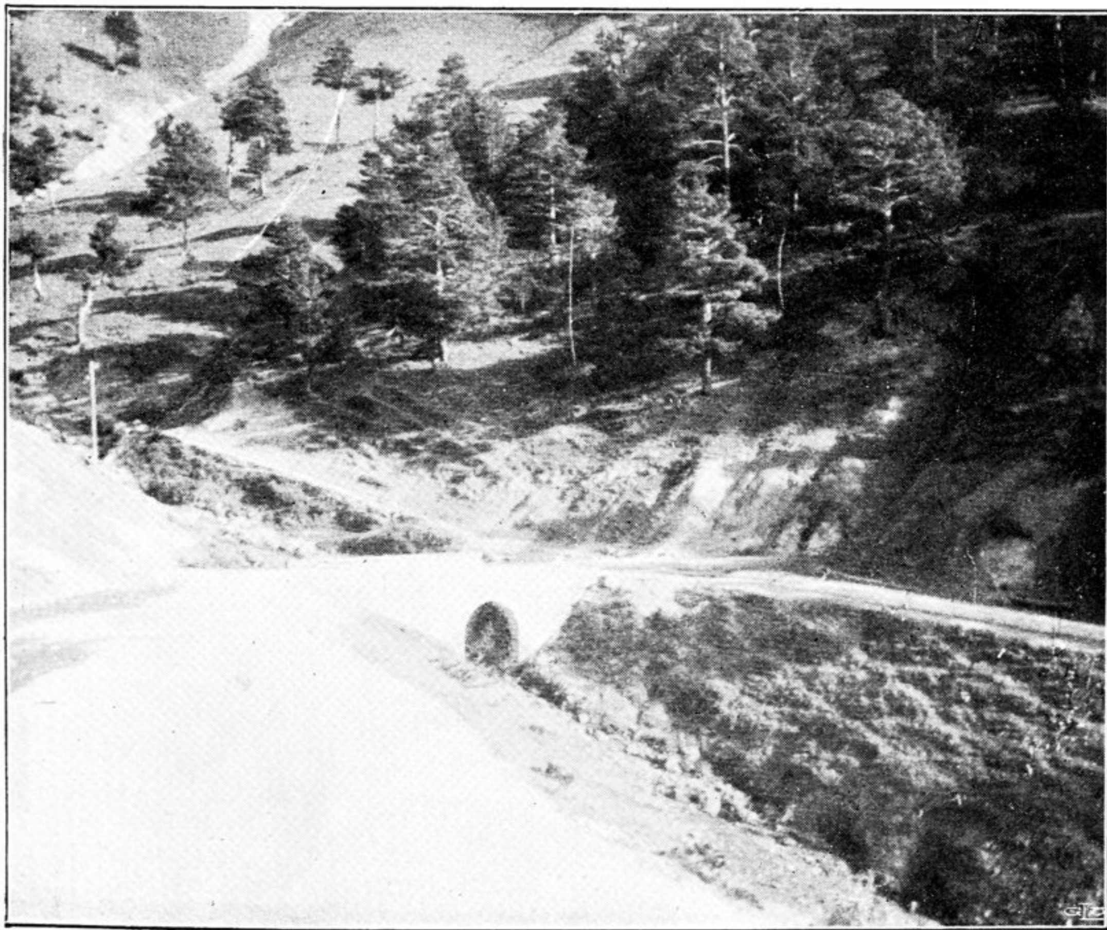
8. STONE BRIDGE WHERE THE ROAD DIVERGES INTO A SIDE VALLEY.
