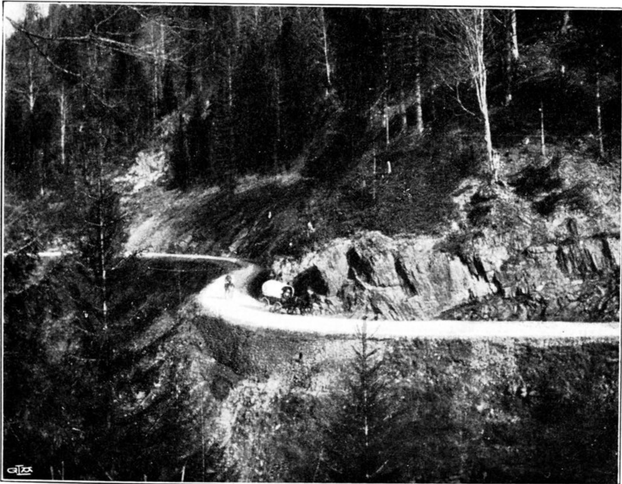
11. ROAD NEAR SIGANA BETWEEN TREBIZOND AND ERZERUM.
