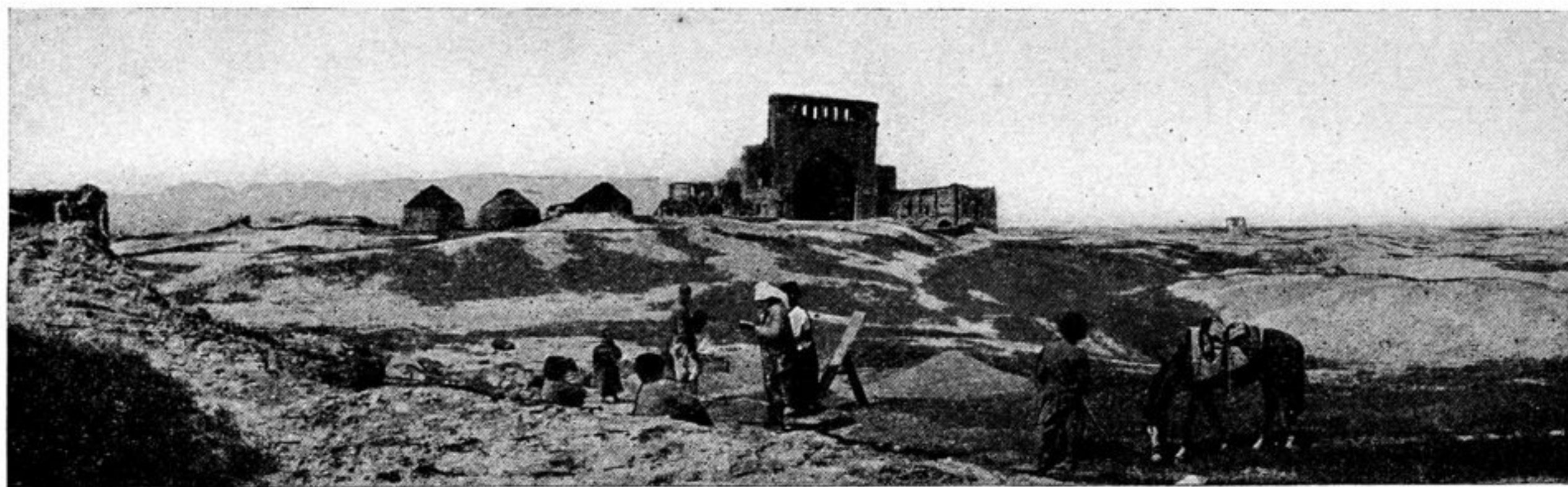
Fig. 16.—Starting a Shaft in the City of Anau.
