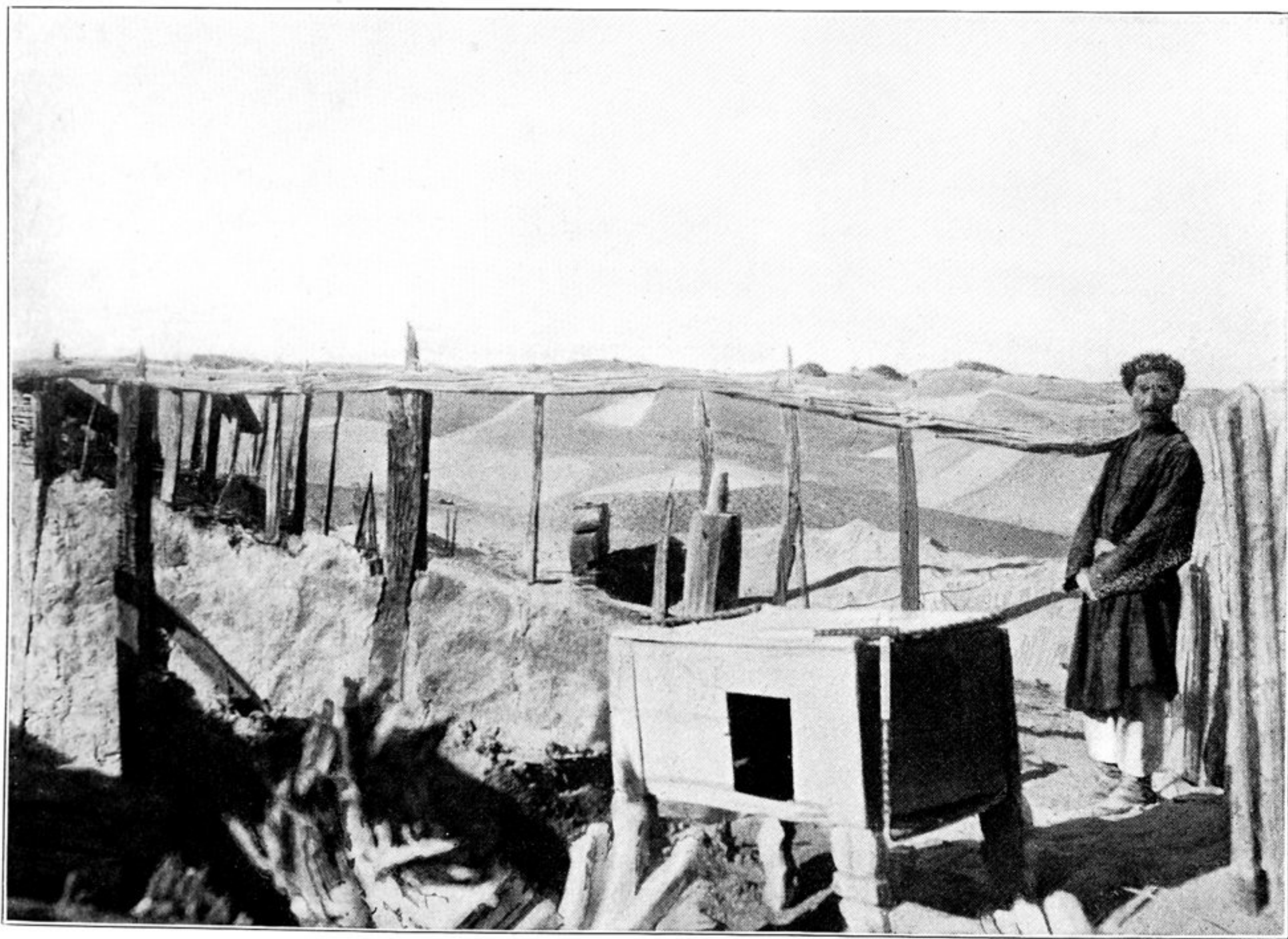
86. ROOM EXCAVATED IN RUIN N. XXVI., NIYA SITE, WITH ANCIENT CARVED CUPBOARD IN WOOD.
