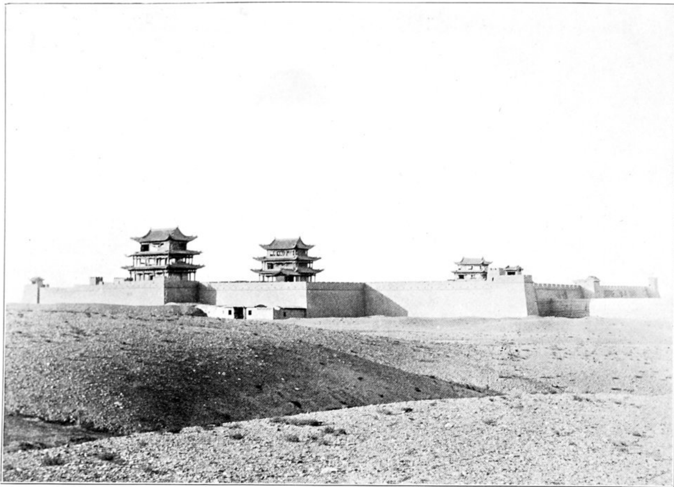
224. THE CHIA-YÜ-KUAN GATE OF THE 'GREAT WALL,' SEEN FROM SOUTH-WEST.
