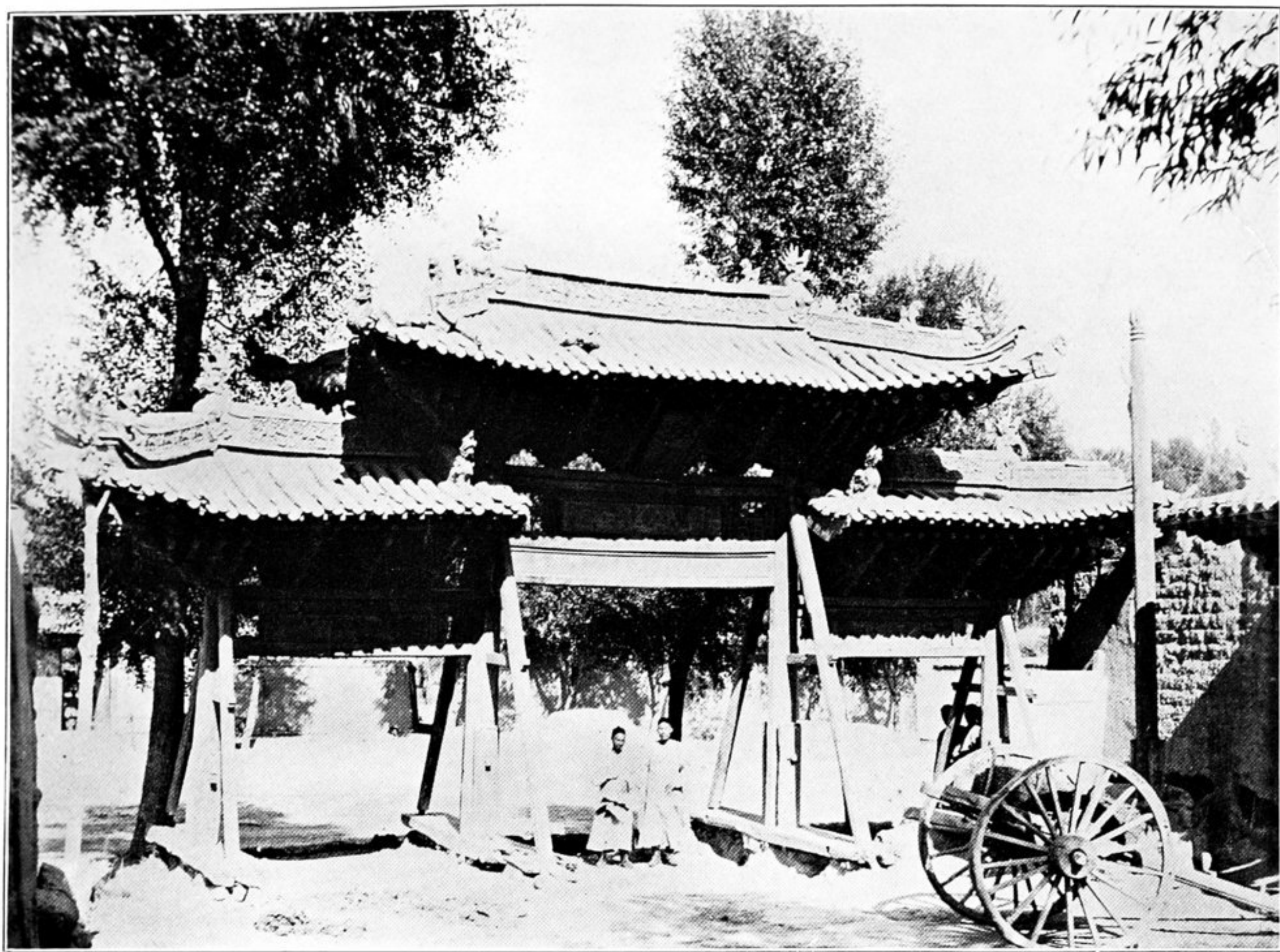
255. MEMORIAL GATEWAY, BUILT ABOUT A.D. 1825, OUTSIDE WEST GATE OF KAN-CHOU.
